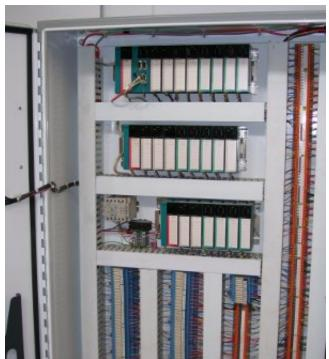
Etheridge Automation has developed an aggregate processing automation system that is modular in nature and can be scaled for the various sizes and configurations of aggregate plants. At the core of the Etheridge Quarry Information Management System<sup>TM</sup> is a SoftPLC programmable controller that communicates over Ethernet to the control room PC. Wonderware Intouch 10.0 is used for the HMI. Etheridge uses SoftPLC because of its reliability, ease of use, processing power and flexibility.
