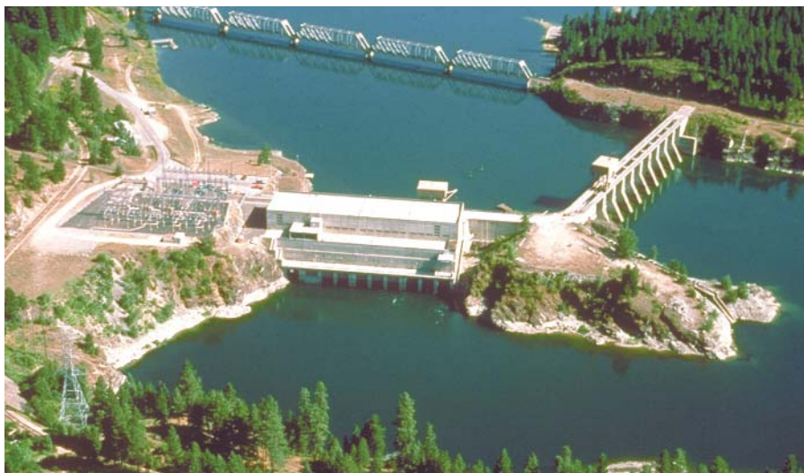
The U.S. Army Corps of Engineers' 43-MW Albeni Falls hydro plant on the Pend Oreille River in Idaho features a new annunciation system for alerting operators and maintenance staff to changes in plant operating conditions.
